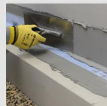
*Embed the MC-FastTape and apply the last waterproofing layer.*
