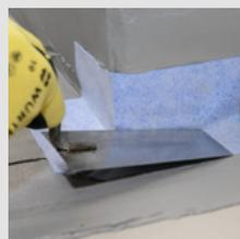
*MC-FastTape AE outer corners or MC-FastTape IE inner corners embedded in the fresh first layer.*
